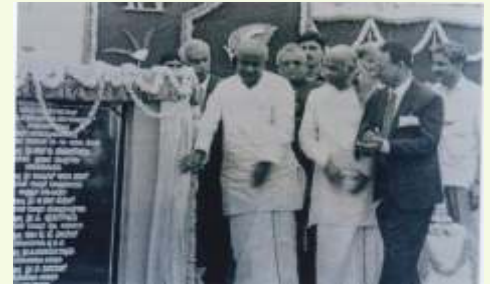
Sri H. D. Devegowda, the then Prime Minister of India laying the foundation stone for construction of Convention Centre
